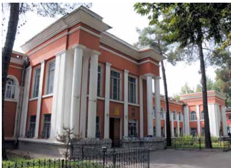
Building of the Institute of Language and Literature of the Academy of Sciences of the Republic of Tajikistan named after A. Rudaki. Earlier, this building was the office of the People's Commissariat / Ministry of Foreign Affairs of the Tajik Soviet Socialist Republic.
